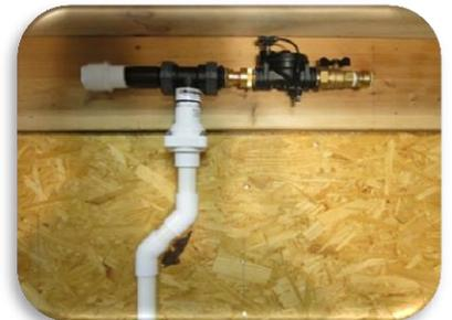
**STEP #3:** Install the discharge pipe using either rigid PVC pipe or the supplied hose or both. {Outdoor discharge shown}
