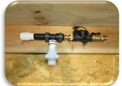
**STEP #2:** Install the suction pipe using either 45 or 90 deg. elbows if necessary.
