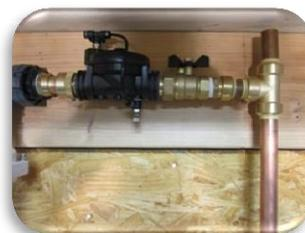
**STEP #6: Install the high water alarm.**
