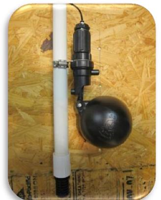
**STEP #5: Connect water line by inserting the tee into a cold water line and pipe to the Basepump.**
