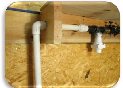
**STEPS #4:** Mount the float valve to the suction pipe and connect the transfer tube.
